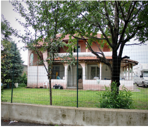
Fig. 11 Two-storey house in the nomad camp of Via Monte Bisbino.
