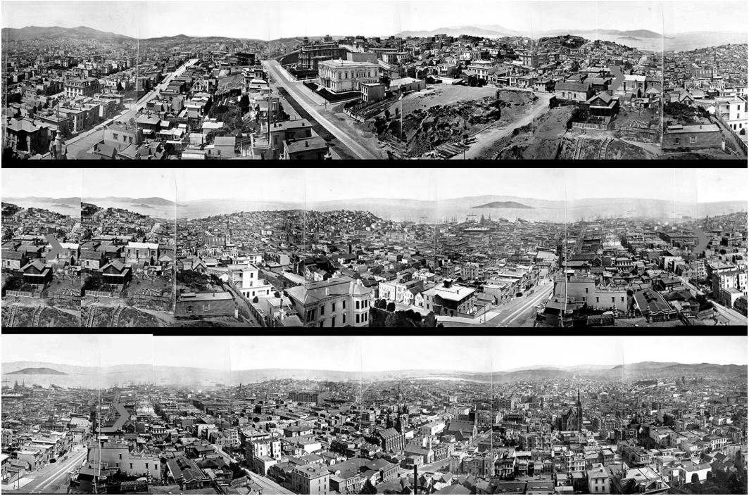
Fig. 10. Eadweard Muybridge, San Francisco , 1877-1980. (Graphic elaboration on the photo by M. Cicala) (Retrieved May, 6, 2023 from https://www.nyhistory.org/blogs/-muybridges-spooky-panorama ).
