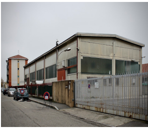
Fig. 8 Example of industrial architecture of the 20 th century.
