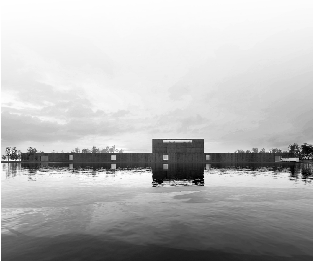
Fig. 1 Alberto Campo Baeza and Raphaël Gabrion, Conservation and Storage Facility for the Louvre Museum in Liévin , 2015. Digital rendering of the building on the lake (Courtesy of Alberto Campo Baeza and Raphaël Gabrion).
